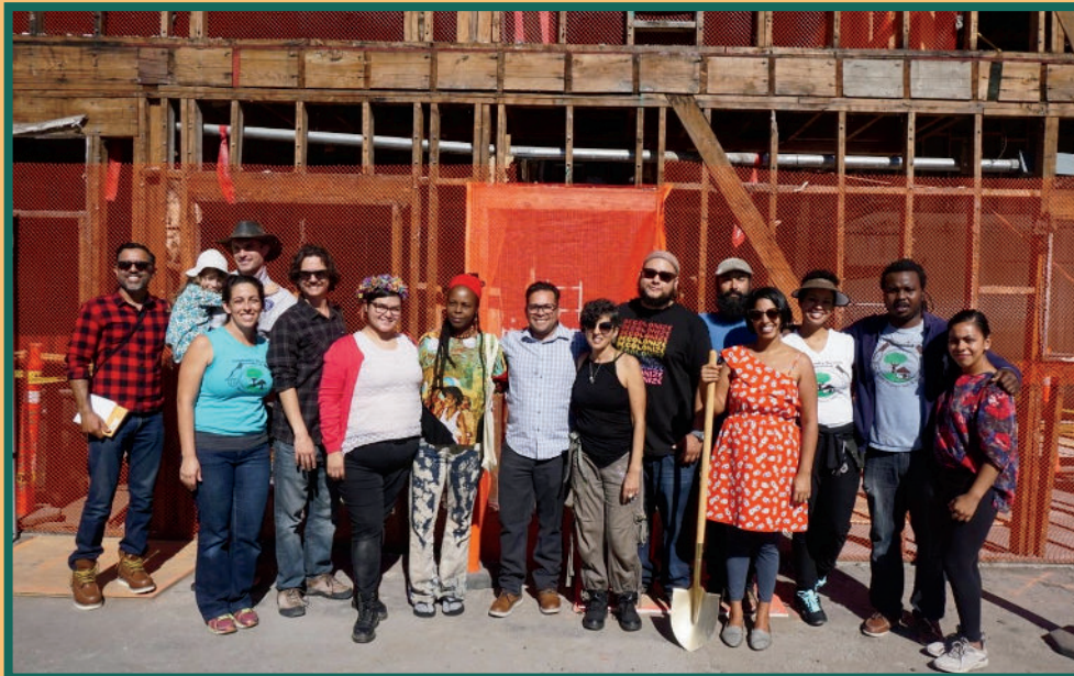
The CSU team at the groundbreaking of the Paul Robeson Community Wellness Center.
